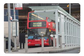
Bollards | Static Manufacturer:ATG Access Standard Tested To: PAS 68:2007 Performance rating: V/7500[N2]/32/90:0/0.0
