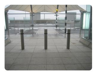
Bollards | Static Manufacturer:ATG Access Standard Tested To: PAS 68:2007 Performance rating: V/3500[N1]/48/90:0/0.0
