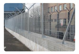
Perimeter Barriers | Vehicle Manufacturer:Britpave Barrier Systems Standard Tested To: PAS 68:2010 Performance rating: V/7500[N3]/80/90:2.5/25.0
