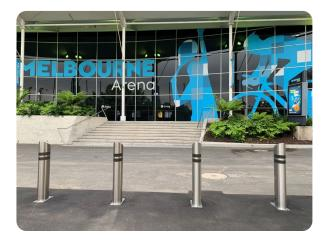
Bollards | Static Manufacturer:Safetyflex Barriers Standard Tested To: PAS 68:2010 Performance rating: V/7500[N2]/48/90:2.8/0.0
