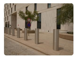
Bollards | Static Manufacturer:ATG Access Standard Tested To: PAS 68:2010 Performance rating: V/7500[N3]/80/90:3.6/7.9
