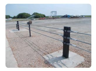
Perimeter Barriers | Vehicle Manufacturer:Safetyflex Barriers Standard Tested To: PAS 68:2010 Performance rating: V/7500[N3]/48/90:3.4/6.4
