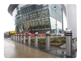
Bollards | Static Manufacturer:Safetyflex Barriers Standard Tested To: IWA 14-1:2013 Performance rating: V/7200[N3C]/80/90:10.5
