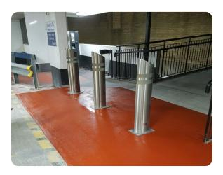
Bollards | Static Manufacturer:Safetyflex Barriers Standard Tested To: IWA 14-1:2013 Performance rating: V/7200[N2A]/48/90:8.2
