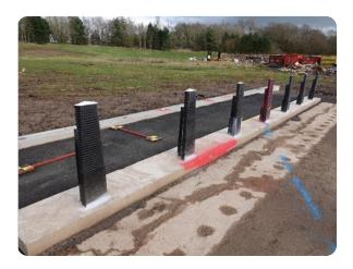
Bollards | Static Manufacturer:Marshalls Standard Tested To: IWA 14-1:2013 Performance rating: V/7200[N2A]/48/30:1.1
