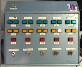
Figure 1: A typical VACP including active VSBs (left); control panel for an active VSB (right).
