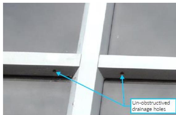
**Figure 1:** Photo showing un-obstructive drainage holes in a window frame.
